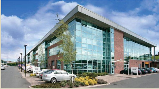
Promoting the development of new employment uses in the unincorporated parts of the county is a major goal of the 2035 General Plan.
